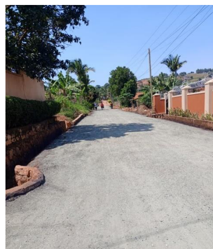
FIGURE 1: SYCAMORE AVENUE TARMACKING
