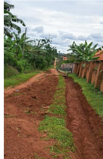
FIGURE 4: MUSIZI ROAD WORKS
